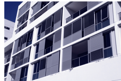
Fig 4: adjustable screens allows provides shading for occupants at different times of the day.
