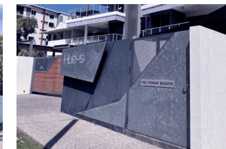
Fig 6: Example of screening to conceal services that is integrated into the overall design of the fence.
