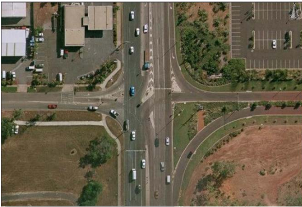
Site 1. Bagot Road – Trower Road
