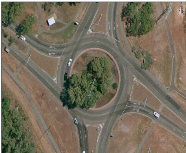
Site 5. McMillans Road – Vanderlin Drive
