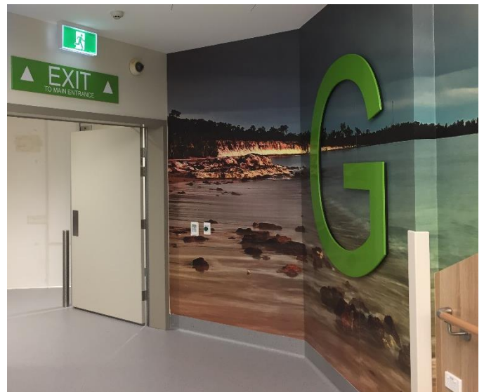
3d image of photographic film applied to wall in lift lobby
