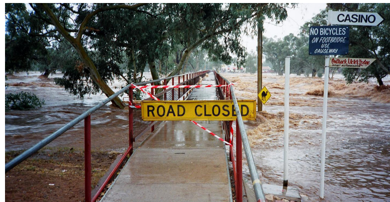
Above: The Todd River flows over the footbridge on Undoolya Road during the 1988 flood.
