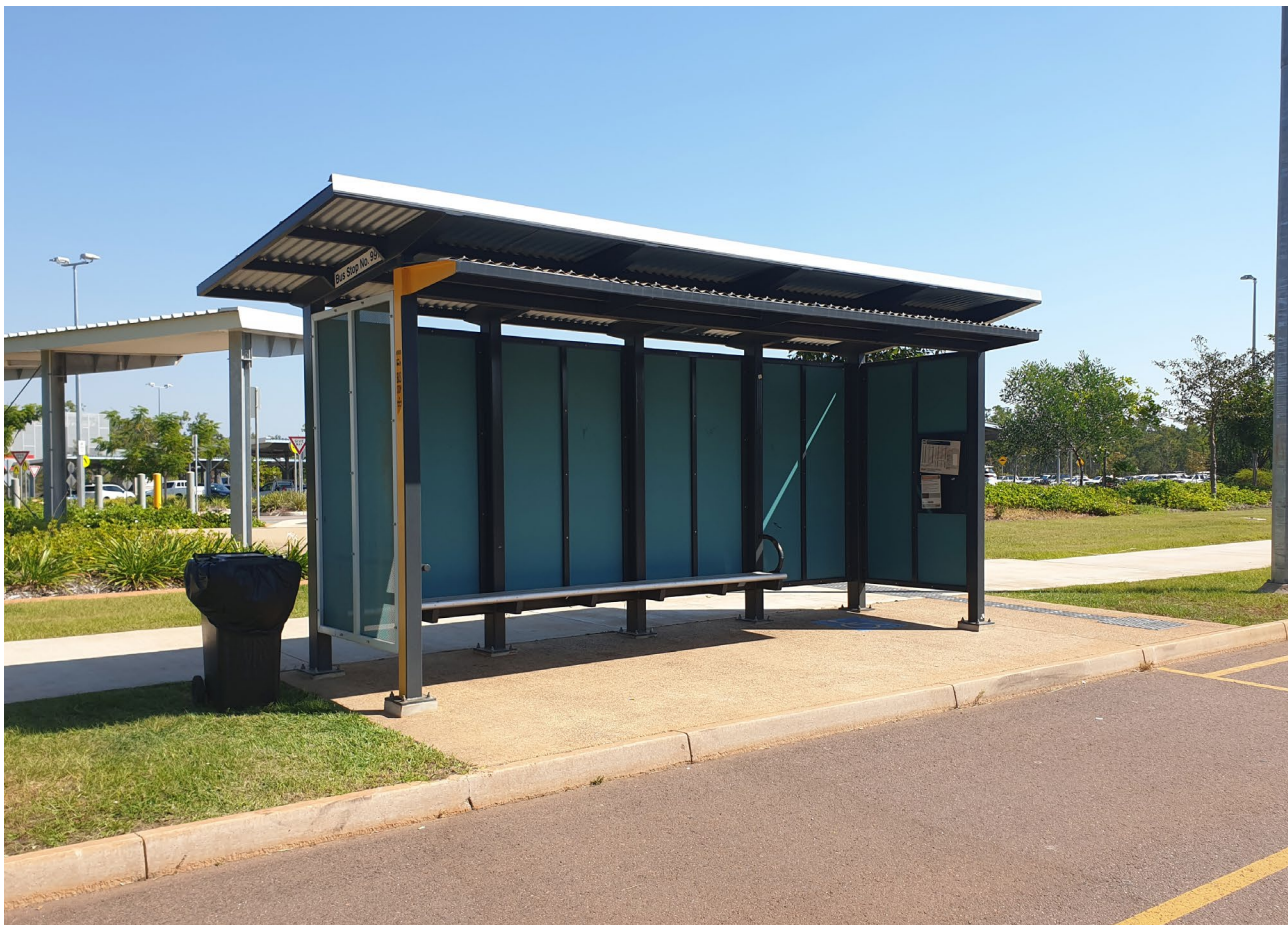
Photo 13: showing an example of a bus shelter Type 14C (4 bays) located near Palmerston Hospital.
