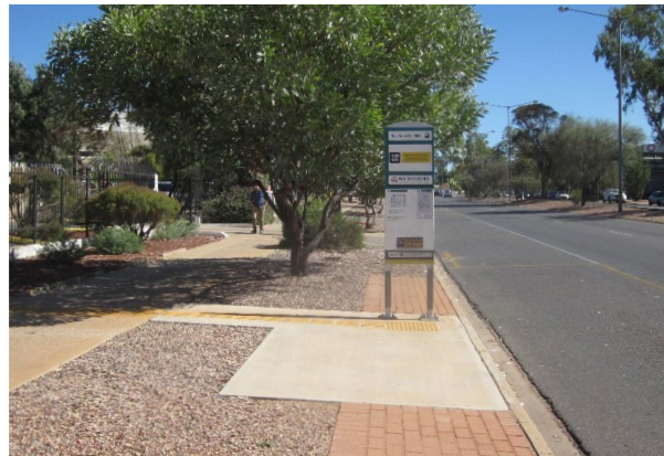
Photo 3: typical supporting infrastructure at a basic bus stop. This stop infrastructure has no seating.*
