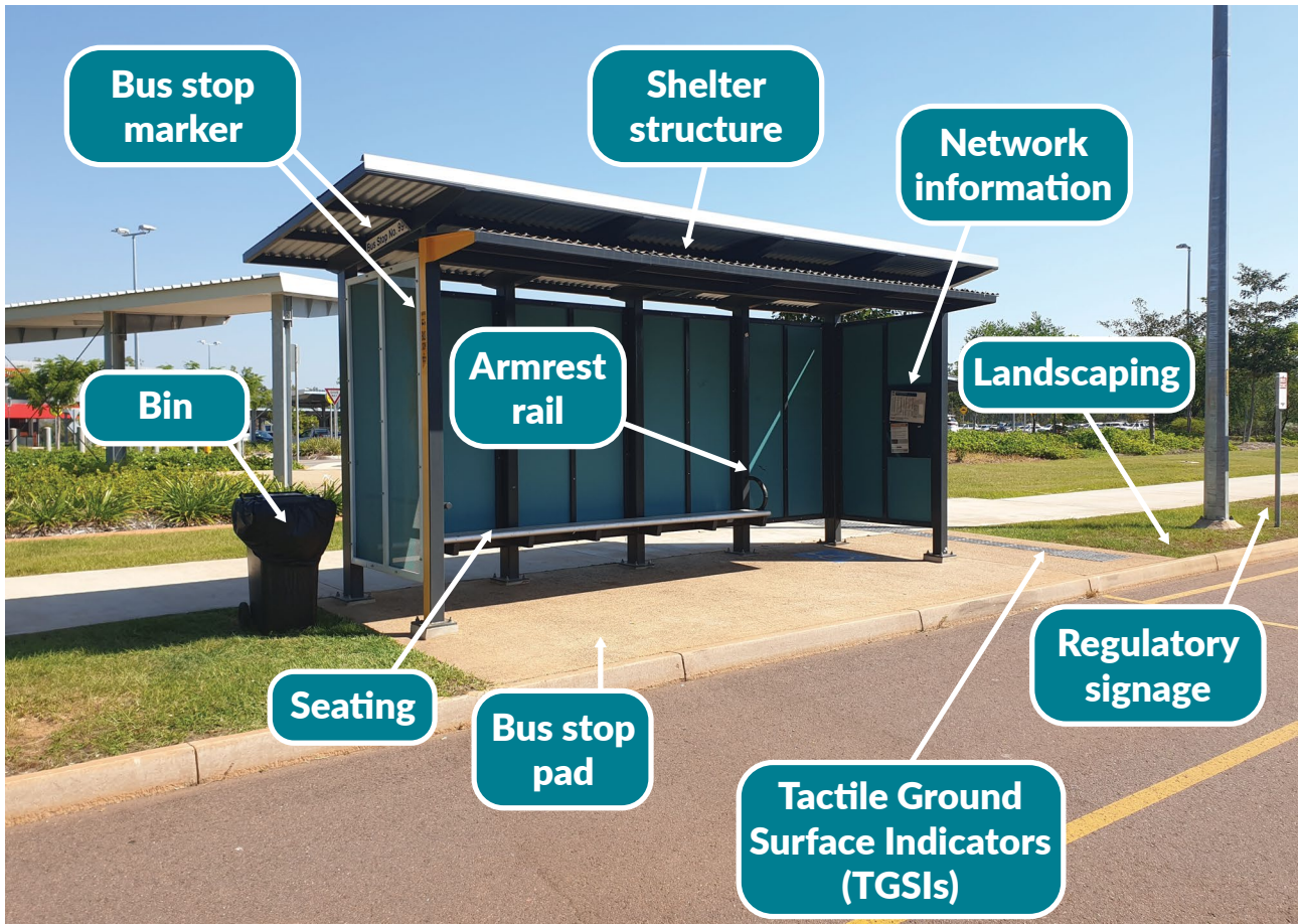
Photo 11: showing some typical components incorporated into bus stop infrastructure.
