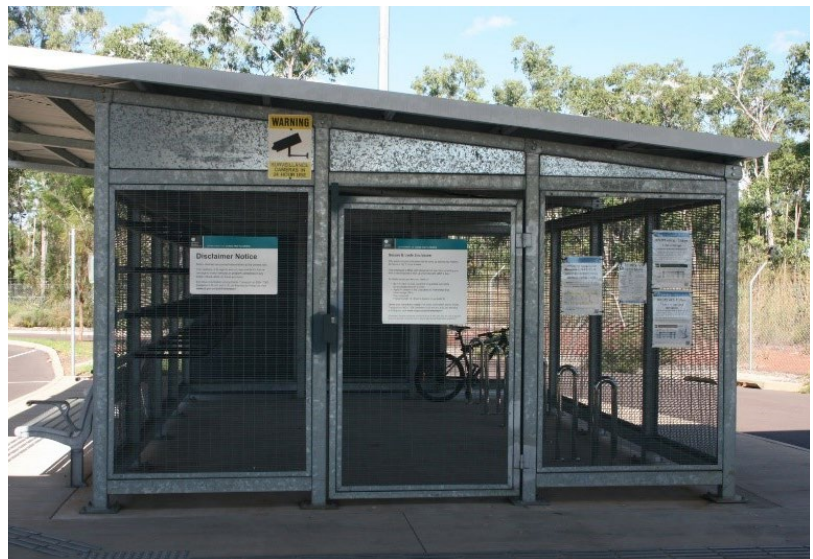
Photo 10: an example of secure bicycle storage facilities and a bus stop shelter installed at Coolalinga Park and Ride.
